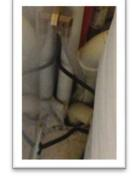
Securely insert the drain hose into your hub drain. Be certain the drain is below the brass outlet fitting on the rear of the dehumidifier. Fasten the hose securely to the wall with a continuous downward slope to the drain (with no bellies or kinks in the hose) so that it cannot be removed from the drain accidentally.
