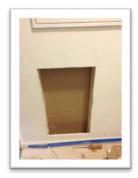
Cut a hole in the sheet rock with a utility knife %" larger than the actual dimensions of the rear of the dehumidifier. Make Sure the opening is square, plumb and offers bottom support for the unit. Opening Dimensions: 14.5"x25.5"x9.38"
