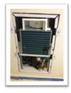
Install 4 screws in mounting flanges, securely into the 2x4 wall studs directly though the sheet rock.
