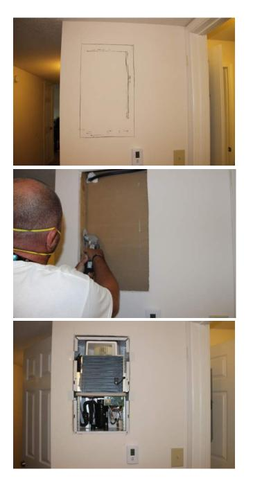
Using a stud finder, we located two 16" W on center studs. A 14.5" X 25.5" template was marked with a 24" bubble level ruler then cut with a vibrating saw. The IW25-1 unit is placed into the wall and secured with 4 wood screws furnished with the unit. A 10' long drain line was attached and inserted into the AHU drain, and
